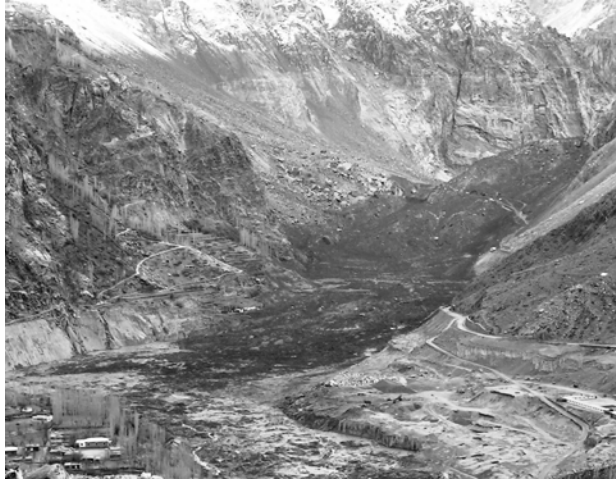
Figure 2. Photograph of the Attabad landslide looking from downstream of the dam. The source area is on the left, and the main landslide mass is on the right side, piled up on the opposite valley wall. The dark mass is the silty-clay mantling the landslide body. The saddle is clearly visible in the centre-right of the photograph.
